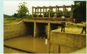
Ranjana-Jharna Sub-Project, Sherpur
