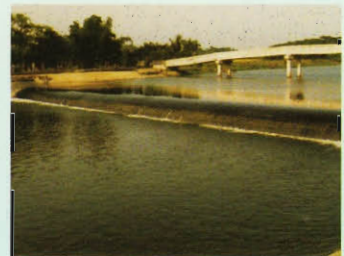
One Rubber dam under operation
